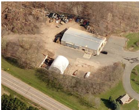
Existing Public Works Facility Site
