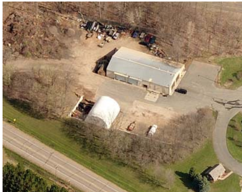
Existing Public Works Facility Site
